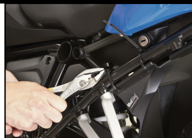
7 After pulling the zip ties as tightly as possible by hand, use pliers to tighten zip ties fully.
